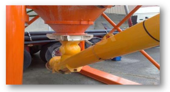
TAKES THE NEEDED CEMENT FOR MORTAR FROM THE SILO TO FEED THE WEIGHING CONVEYOR . WAM BRAND. 8'(Ø219 mm ) MOTOR POWER IS 9,2 Kw. SILO CONNECTION POINT IS MOVABLE.
