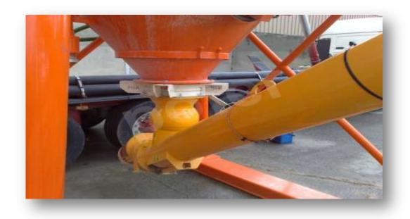
TAKES THE NEEDED CEMENT FOR MORTAR FROM THE SILO TO FEED THE WEIGHING CONVEYOR. WAM BRAND. 8'(\$\psi^2\$19 mm) MOTOR POWER IS 9,2 Kw. SILO CONNECTION POINT IS MOVABLE.
