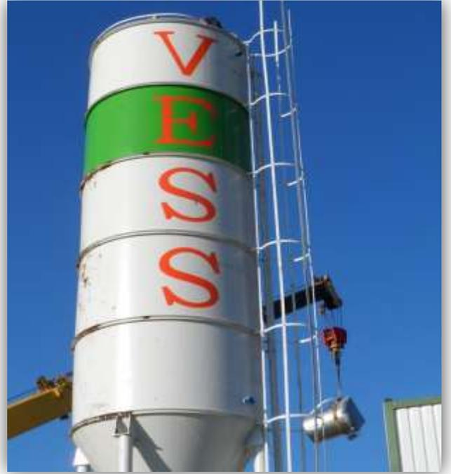
CEMENT STORAGE EQUIPMENT. BESIDES ARE WALKING STAIRS FOR EMERGENCIES. THE CAPACITY IS 200 TON AND REPLACEABLE CARTRIDGE FILTER IS PROVIDED. THERE IS ALSO 2 PIECES LEVEL MEASURING CENSOR PROVIDED AND SAFETY VALVE TO PREVENT OVERFILLING. TO DISCHARGE THE SILO INTO THE CEMENT FEEDING SCREW THERE IS A WAM BRAND VALVE. MANUFACTURED AS STEEL CONSTRUCTION USING 5 /6 mm. SHEET METAL.
